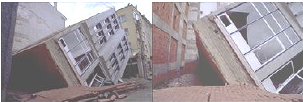
Figure 1: Liquefaction induced bearing capacity failure in the Kocaeli earthquake (Photo courtesy NISEE website, University of California, Berkeley).
