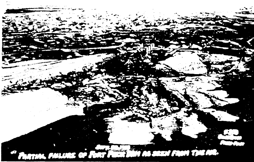
Figure 8. Partial failure of Fort Peck Dam as seen from the air.
