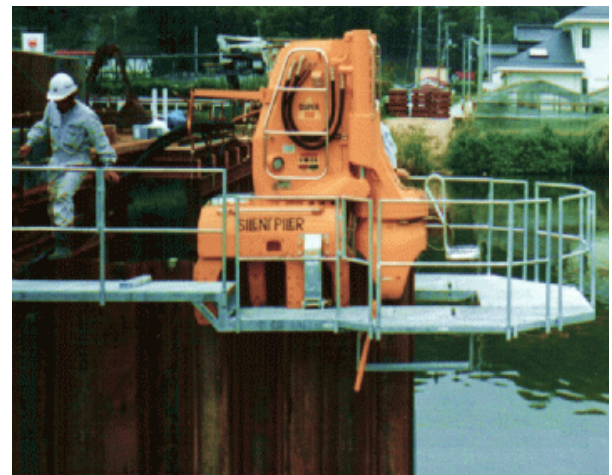
Figure 1.1: A press-in pile driver
