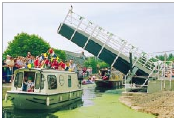
Fig. 8: Bonds Mill Lifting Bridge
