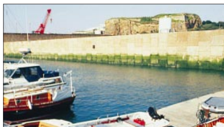
Fig. 11: Wall in tidal zone reinforced with polyester strips
