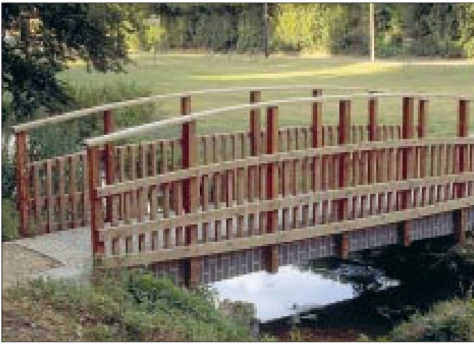
Fig. 3: Tring Footbridge: prestressed masonry
