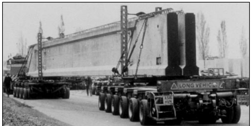
Fig. 3. Transportation of a pair of precast beams by road
