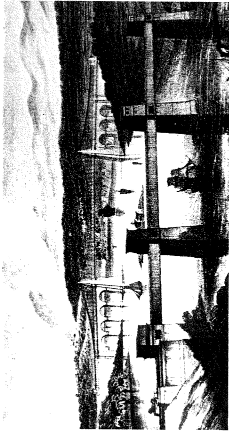
Figure 6 Two different designs in the Menai Straits in North Wales: the Menai Suspension Bridge (foreground) and the Britannia Tubular Bridge.
