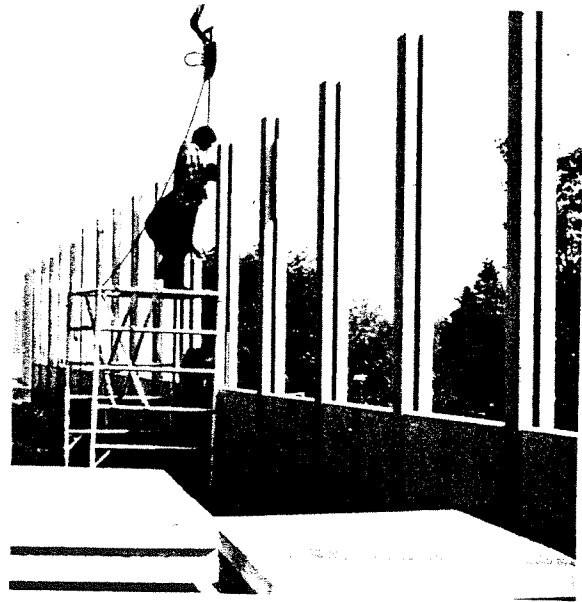
Figure 44.5 Noise barrier posts pretensioned with Arapree tendons. (Courtesy of Akzo)
