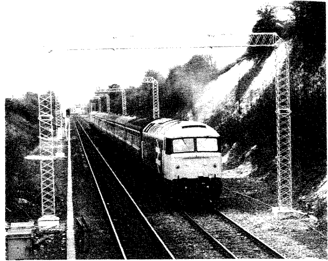
Fig. 11.2. British Railway electrification gantries (courtesy BP Advanced Materials Ltd)
