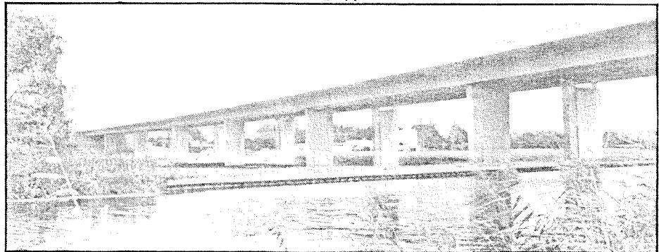
Figure 10: Exe Viaduct (photo Freeman Fox and Partners)
