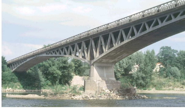
Figure 1: Boutiron Bridge, Vichy
