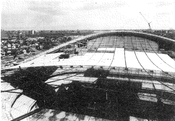
Figure 17. Calgary Saddledome under construction
